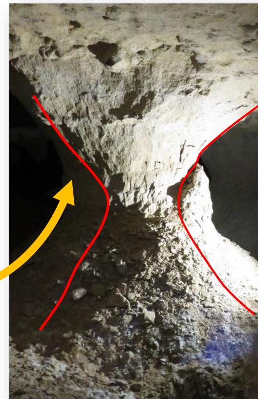
Photo of slender pillar from Malogne underground quarry
