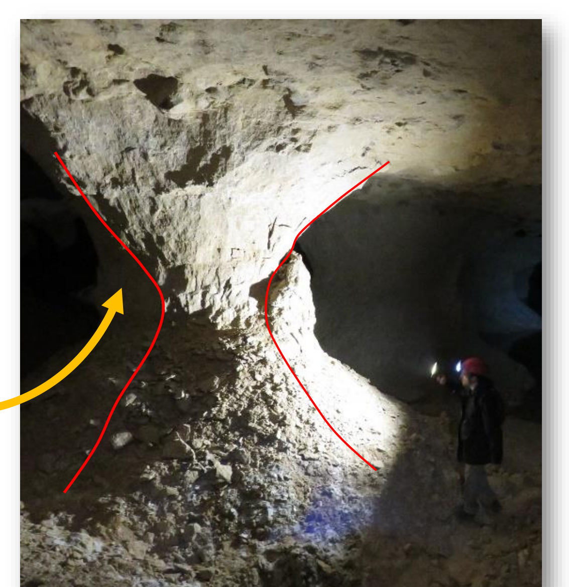
Photo of spalling pillar from Malogne underground quarry
